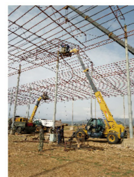
徐工伸缩臂叉装机海外搭建钢结构 XCMG Telescopic Handlers Build Steel Structures Overseas
