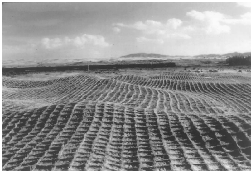
Figure 1. Straw checkerboards are used to fix moving sand dunes along the railway of Baotou–Lanzhou in Shapotou, Tengger Desert.
