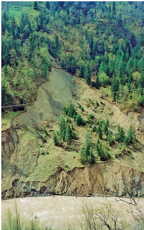
Fig. 1. A slump block breaking away from the riverbank and irreversible loss of loose slope sediments. The Adjaritskhali River, Mountainous Adjara, Georgia
