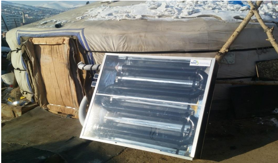
Figure 3. Actual air heating collector
