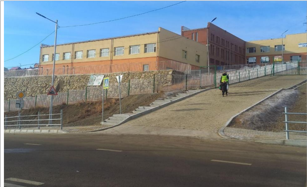
A front view of the school building
