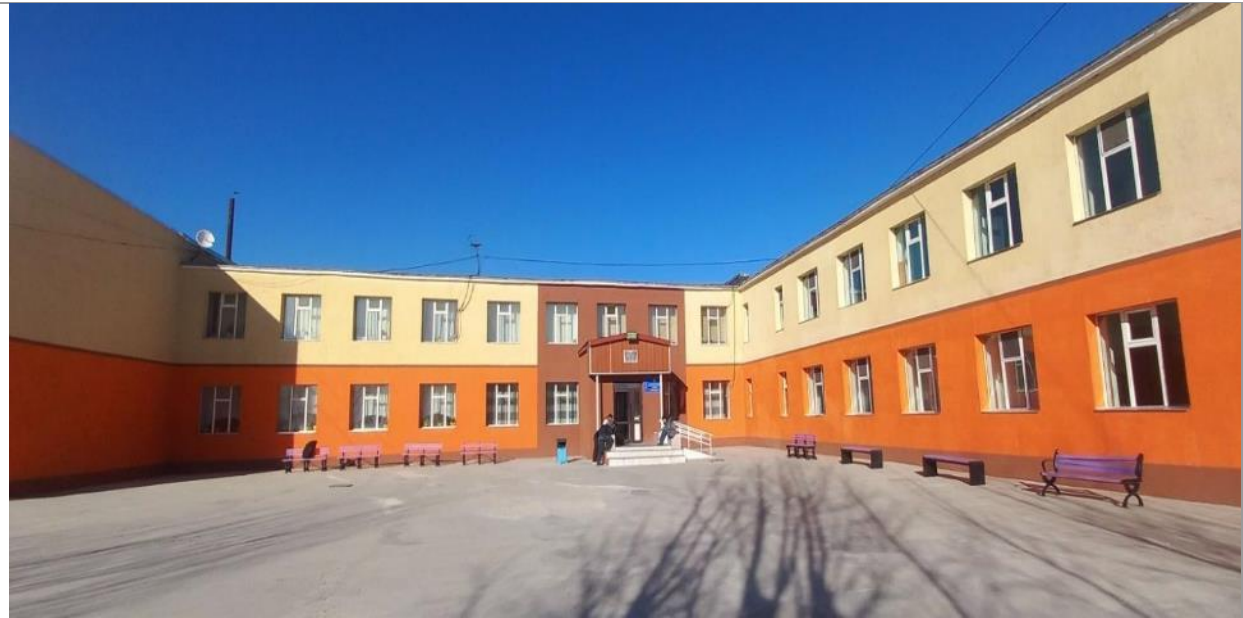
A front view of the school building
