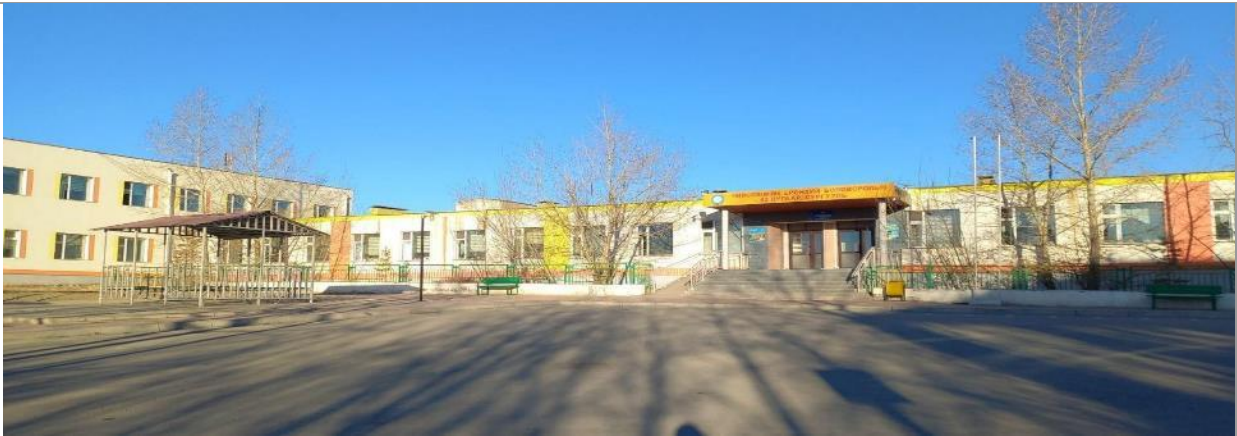
A front view of the school building
