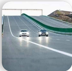
204.6 km of Darkhan-Ulaanbaatar highway
